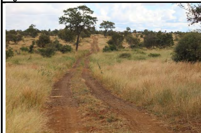
Figure 3: Access Road: Mitre drains have been slashed. Monitor to ensure adequate run-off.
