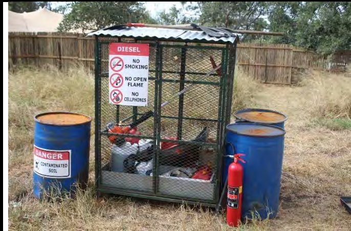
Figure 9: Hazardous Liquids: Locked and stored on a bund separately.
