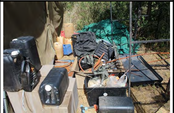
Figure 30: Redundant Materials and Equipment: Remove off site.
