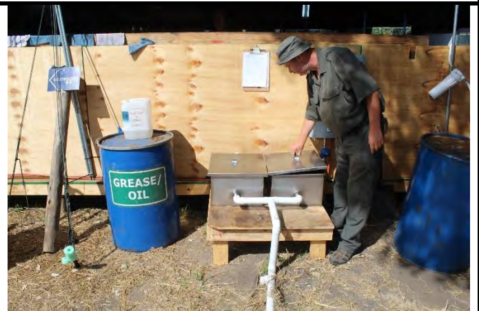
Figure 22: Waste Management: Grease traps are functional.
