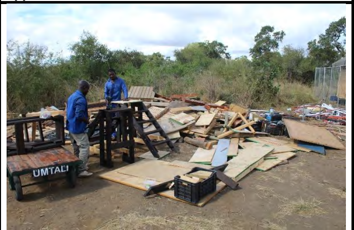
Figure 28: Redundant Materials and Equipment: Remove off site.
