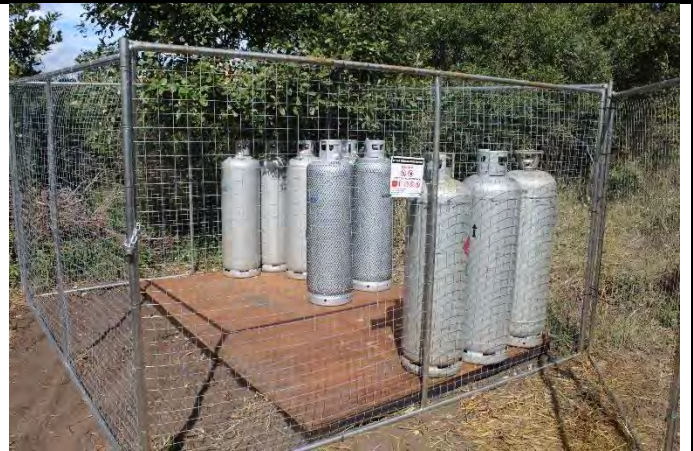
Figure 10: Gas Cage: Locked and stored separately.
