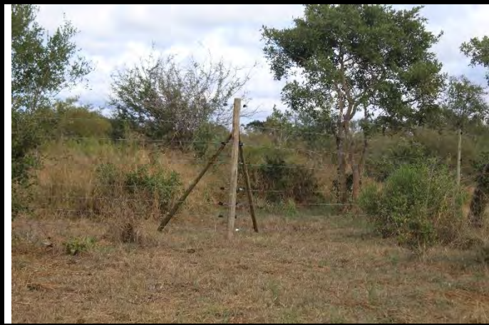
Figure 13: Perimeter Fence: Functional and electrified.
