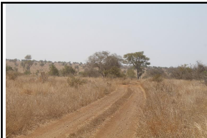
Figure 1. Access Road: Stable. Monitor to ensure adequate run-off.
