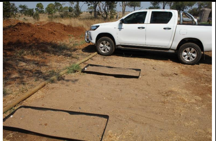
Figure 10: Drip Trays: All vehicles are parked over drip trays. Good.
