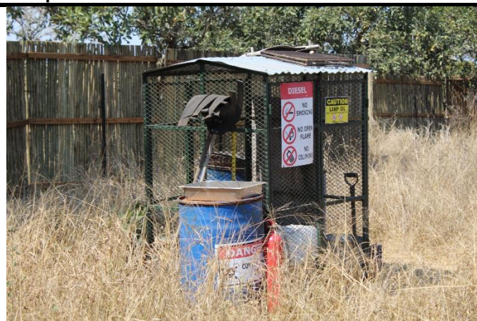
Figure 4: Hazardous Liquids Storage Cage: Locked and stored separately.
