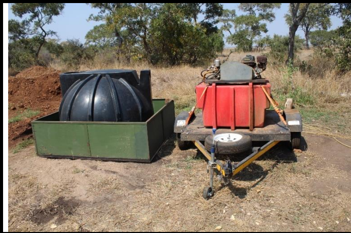
Figure 19: Sewerage Collection Tank and Fire Fighting Equipment: Functional and stored in a dedicated location.
