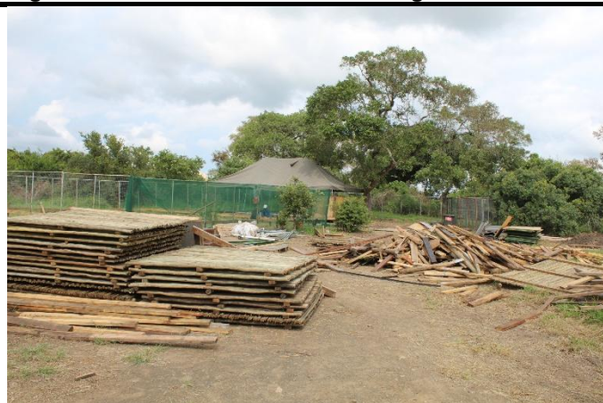
Figure 10: Kitchen and Back of House Area: Being established.
