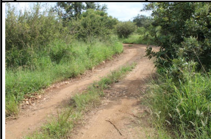
Figure 9: Access Road: More speed humps and gravel is added where applicable.
