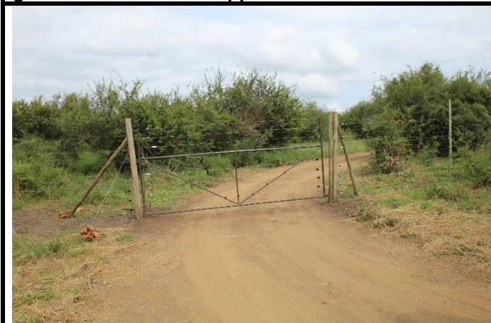
Figure 11: Perimeter Fence: Erected to ensure staff safety during site establishment.
