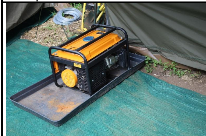
Figure 5: Mobile Generator: On a drip tray. Good.
