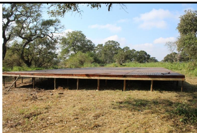
Figure 20: Guest Facilities: Being installed.
