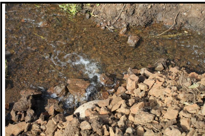
Figure 7: Access Road: Drainage pipes have been installed. Water flow is still ongoing.
