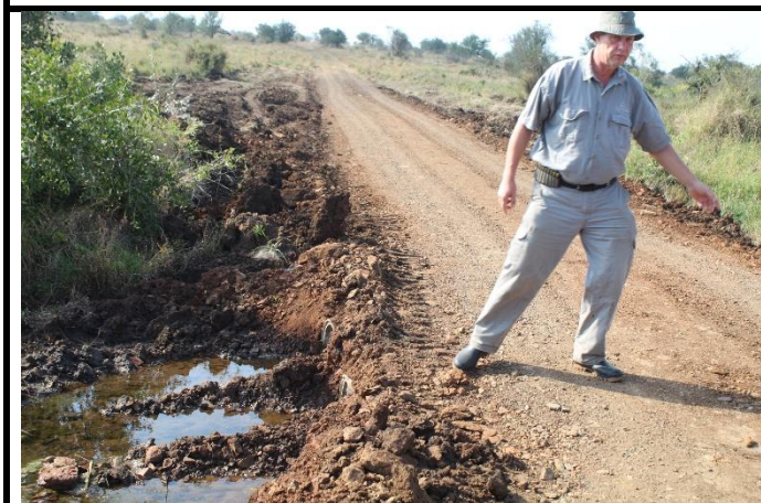
Figure 5: Access Road: Drainage pipes have been installed. Good.
