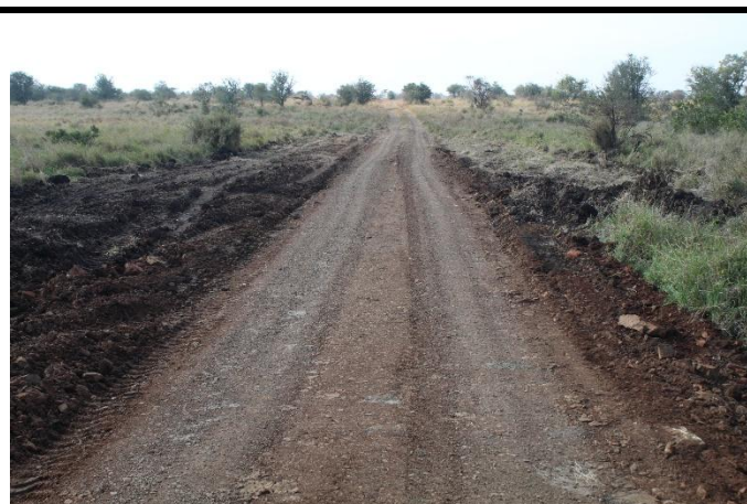
Figure 2: Access Road: Shape the roadside verges to fit in with the lie of the land.
