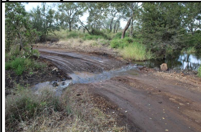
Figure 11: Drainage Line near the Camp: Pipes must be installed as per specifications to ensure ongoing drainage.
