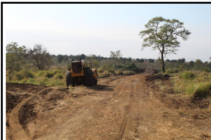
Figure 1. Access Road: Shape the roadside verges to fit in with the lie of the land.
