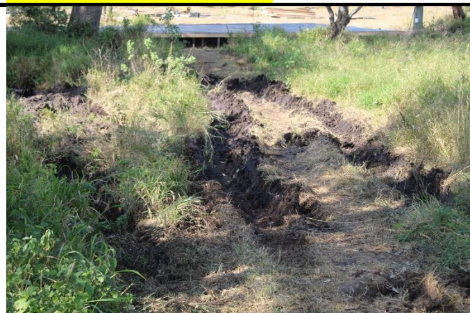
Figure 4: Inside the Camp: Repair and rehabilitate the damage caused by vehicle tracks inside the camp.
