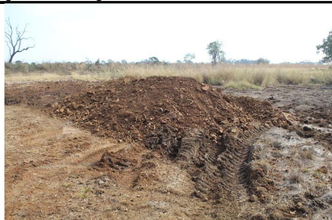
Figure 10: Gravel Stockpile: The final section of the access road near the camp still requires attention.
