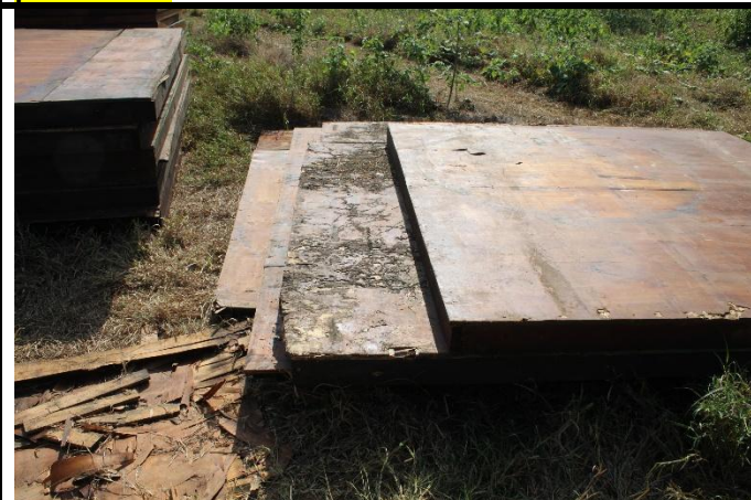
Figure 18: Guest Floorboards: Several boards have been damaged.
