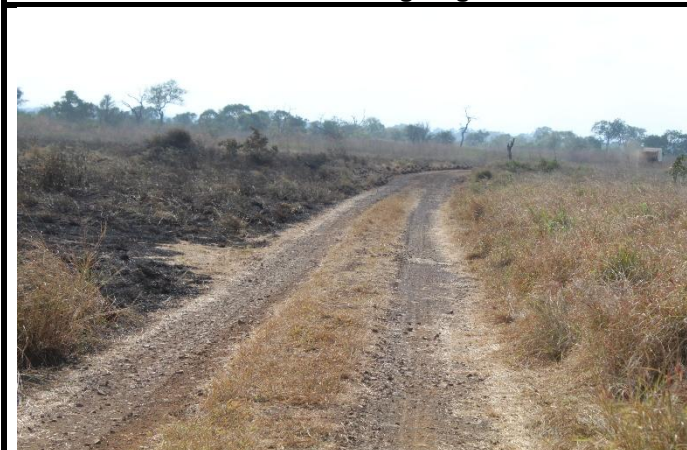
Figure 9: Access Road: Several sections have been graded and or gravel has been added. Good.
