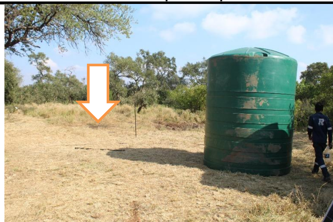
Figure 12: Perimeter Fence: Not completed yet. Should have been erected before staff stayed on site.
