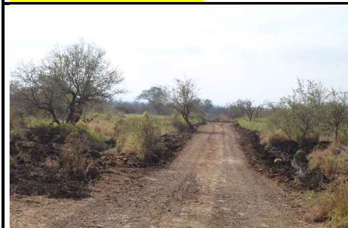
Figure 3: Access Road: Shape the roadside verges to fit in with the lie of the land.
