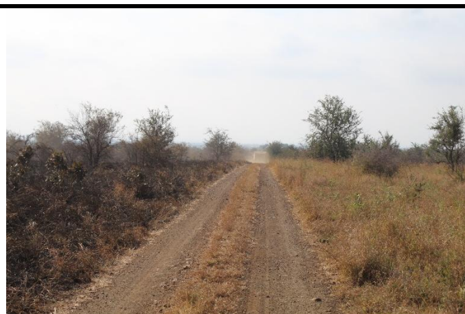
Figure 8: Access Road: Several sections have been graded and or gravel has been added. Good.
