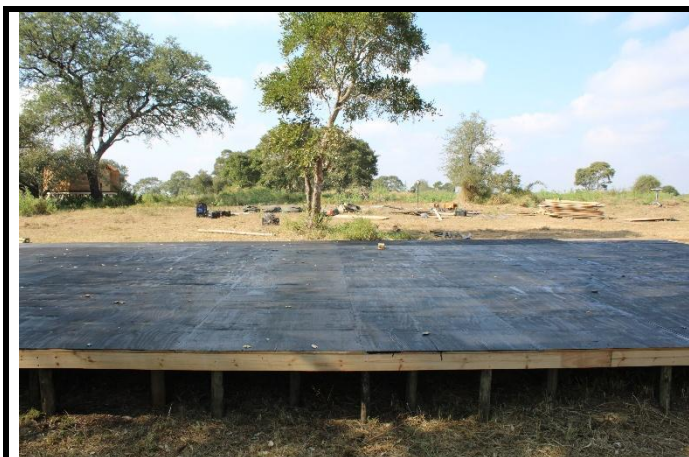
Figure 19: Guest Facilities: Being installed.
