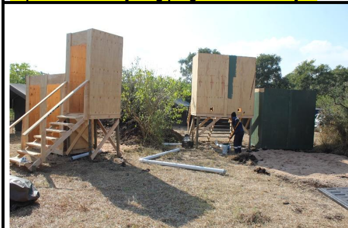
Figure 17: Staff Ablutions/Showers: Being installed.
