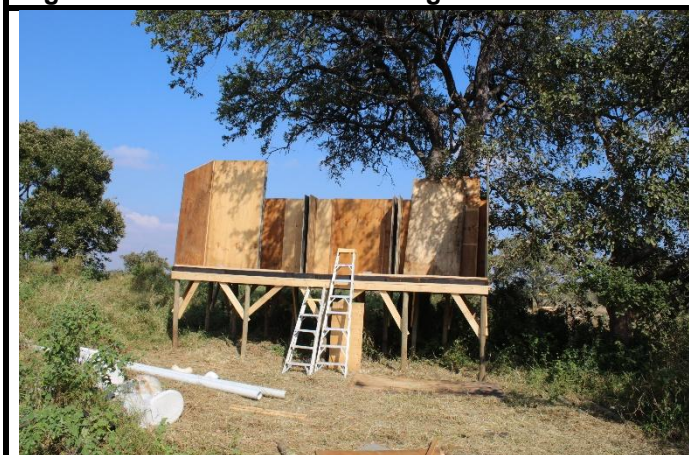
Figure 21: Guest Toilet Facilities: Being installed.
