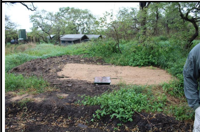
Figure 9: BOH Soak Away: Will be replaced by a septic tank in 2027.
