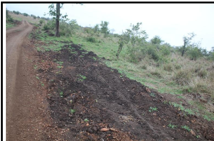
Figure 1. Access Road: Shape the roadside verges to fit in with the lie of the land. Repeat from Audits Nr. 9 and 10.
