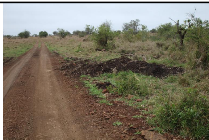
Figure 2: Access Road: Shape the roadside verges to fit in with the lie of the land. Repeat from Audits Nr. 9 and 10.
